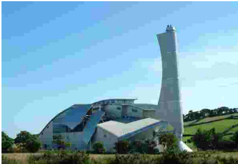
Figure 34: An incinerator on the Isle of Man 27
